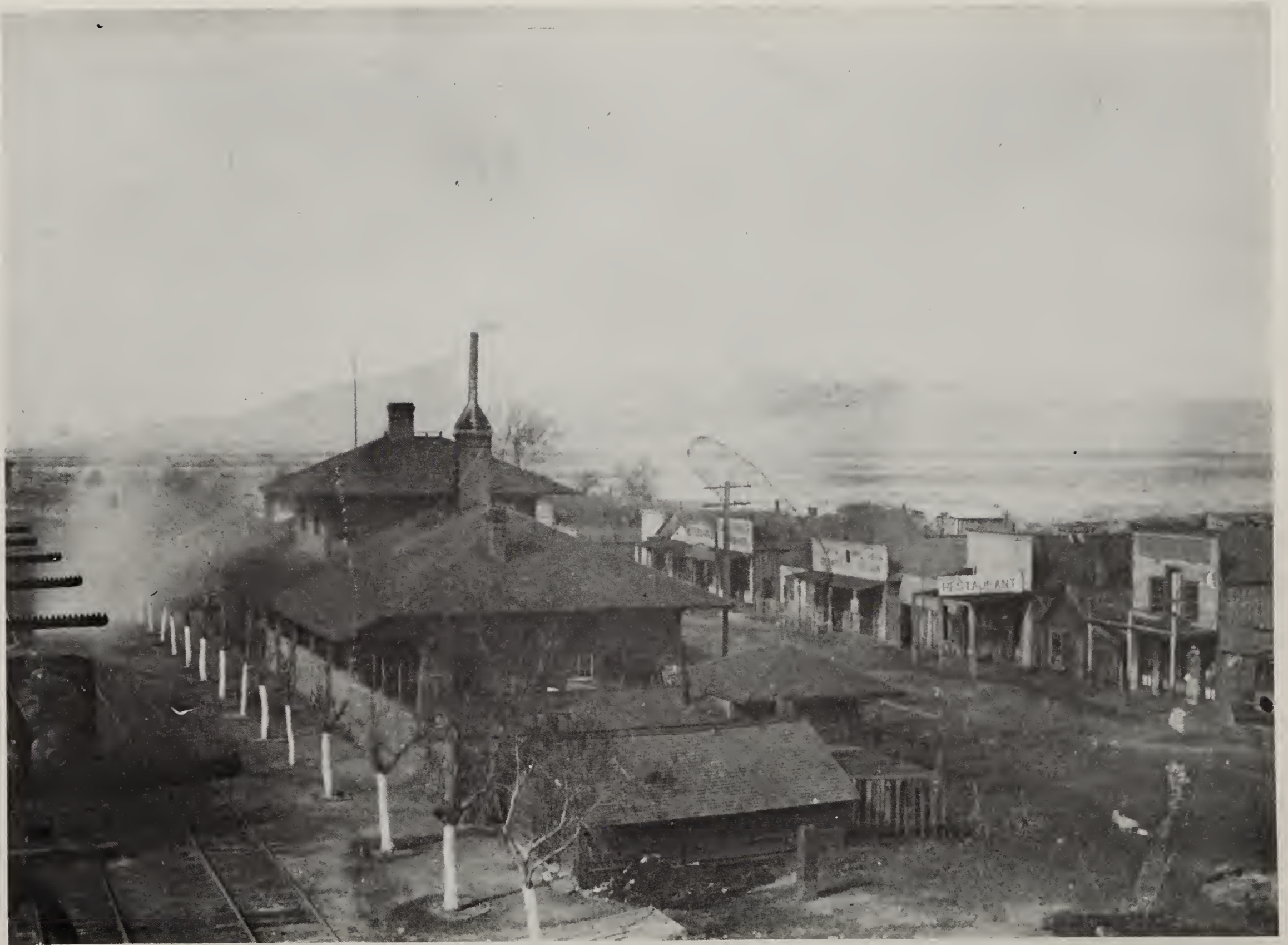
Figure 32: Terrace railroad depot and mainstreet ca. 1880 (courtesy of Southern Pacific).
